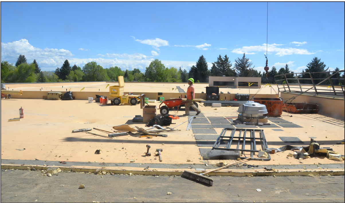
A Pocatello Roofing crew replaced the leaking roof over the Willow Creek badging office early this summer.
